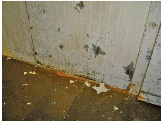
Figure 1. Damaged and corroded steel sandwich panels.
