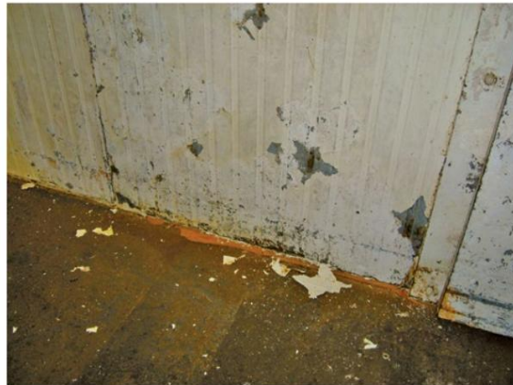
Figure 1. Damaged and corroded steel sandwich panels.
